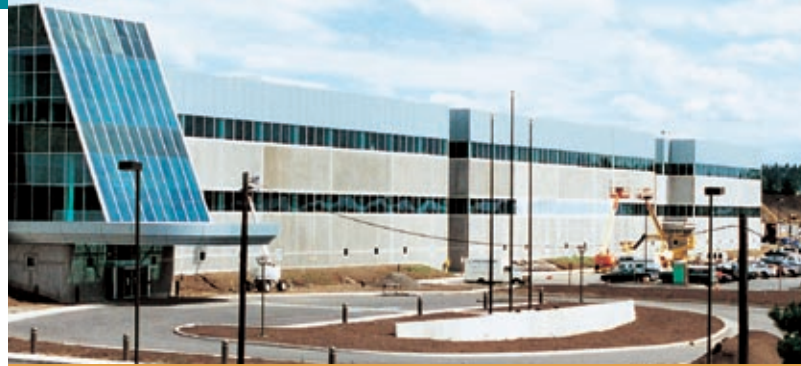
Shin-Etsu Handotai America, Inc. is investing US$710 million to expand and upgrade its facilities. CZ single crystal production for 8-inch wafers has already begun.
