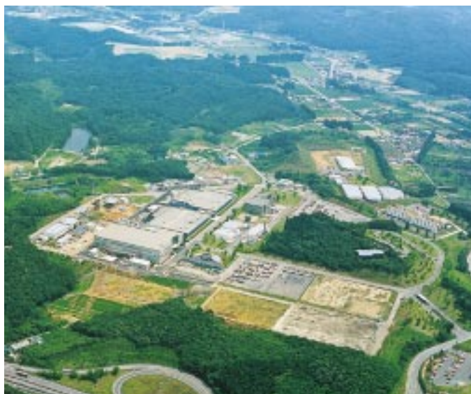
Shin-Etsu Handotai's Shirakawa Plant, Shin-Etsu's first facility to have earned ISO 14001 certification, a new international standard for environmental management.
