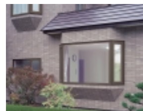
PVC is used in sash has superior heat-retention capabilities and durability against corrosion and climate.
